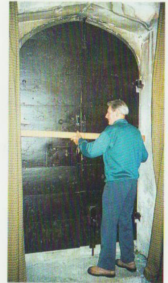
Westwood St Mary's doors are still secured against intruders by a traditional wooden bar
