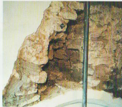
A close-up of the exposed rubble consisting of large weathered lumps of stone
